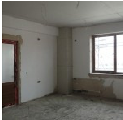
A corridor and a room in the newly built
